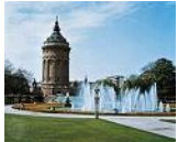
Water Tower - Mannheim Landmark
